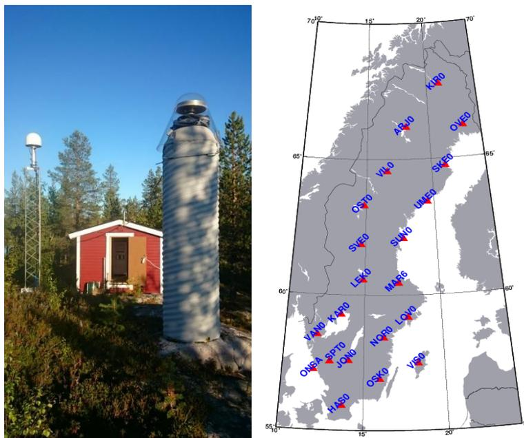
All 21 mast stations at the fundamental sites, except one, were installed in 2011 (ONS1 was installed in January 2012). The close-by truss mast stations are mostly within 10 meters distance from the pillars and at approximately the same height. They are equipped with individual calibrated Leica 3D choke ring antennas with belonging radome (LEIAR25.R3, LEIT). The plan was to let the masts take over
